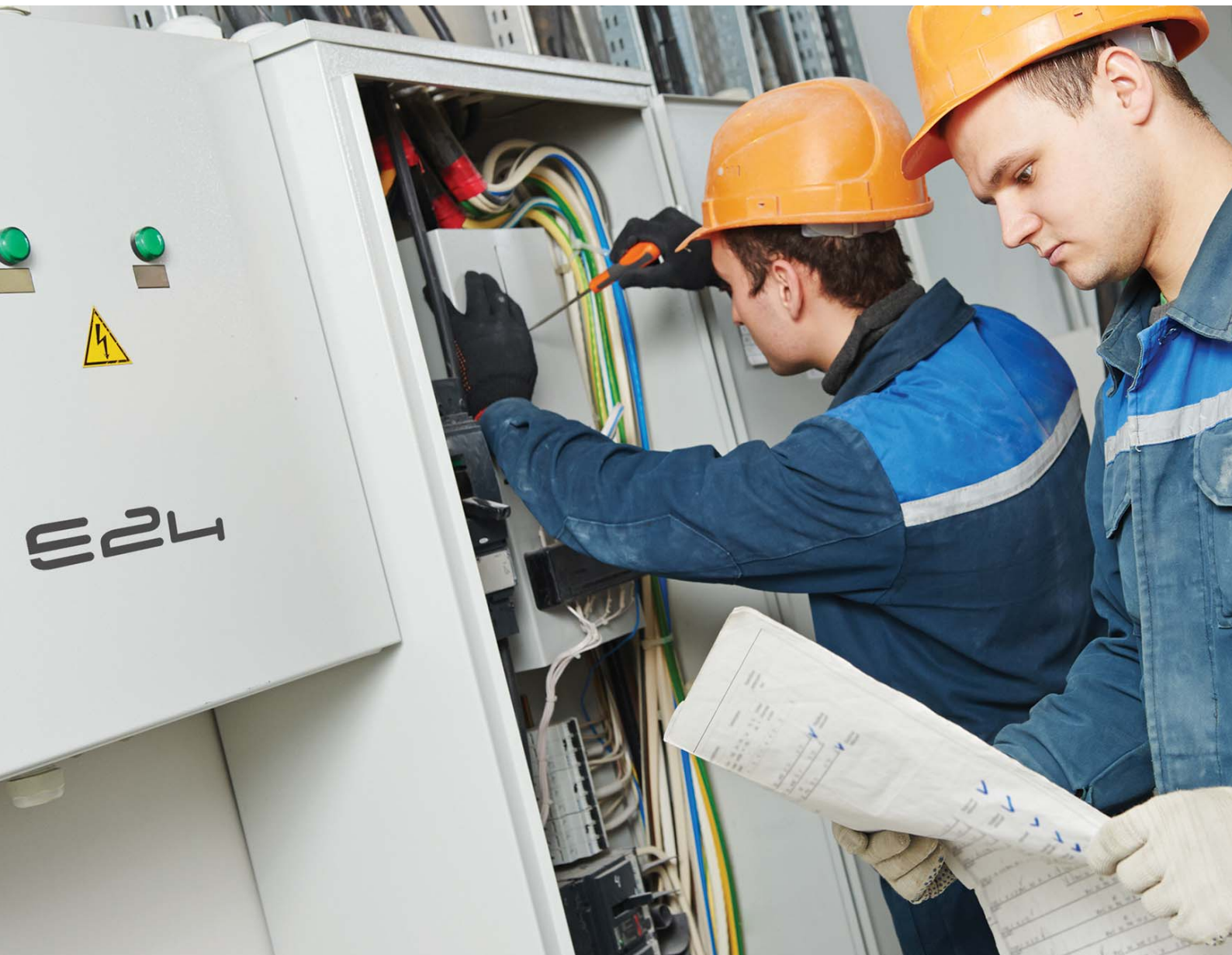
E24 technicians commissioning a new system.
